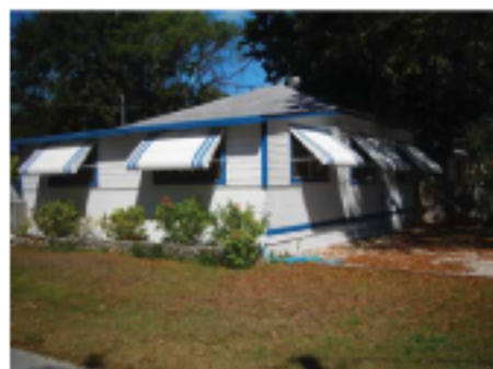
149 Sunrise Drive Façade Facing North of Northwest
