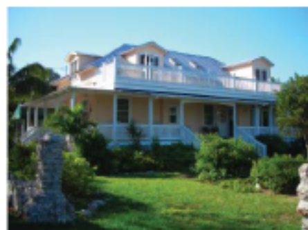
200 Beach Road Facing Northwest
