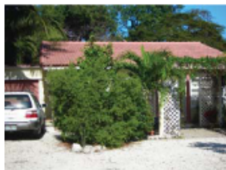
115 Coconut Row Facing North-Northeast
