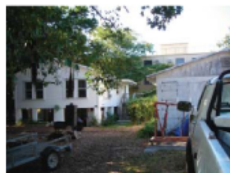
204 Ocean Boulevard Facing Northwest
