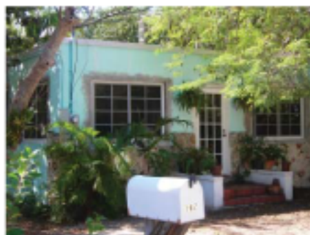
162 Sunrise Drive Façade Facing South
