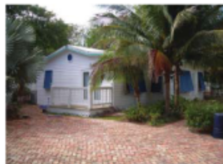
114 Lowe Street Facing Southwest
