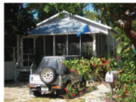
181 Lowe Street Facing North
