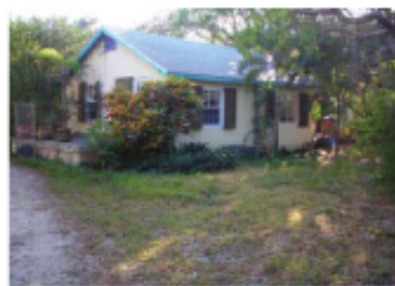
178 Beach Road Facing Northwest.
