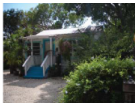
124 Lowe Street Facing South
