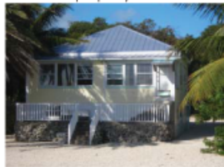
256 Tarpon Street Façade Facing West
