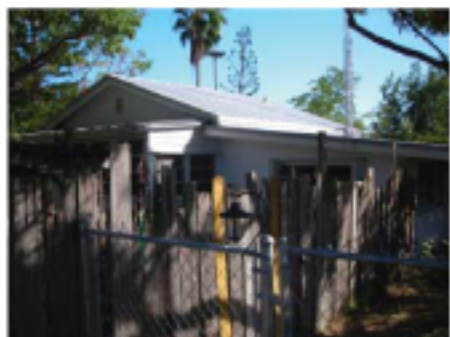
240 Lincoln Avenue Facing Southeast
