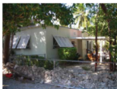
195 Lowe Street Facing North
