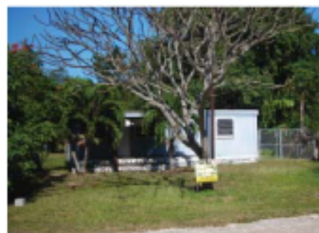
129 Coconut Row Facing Northeast
