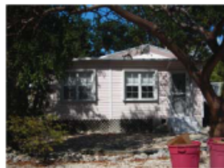
Facade of 185 Lowe Street Facing North
