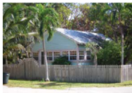
180 Lowe Street Facing Southeast
