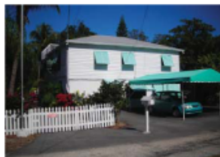
139 Coconut Row Facing Northeast
